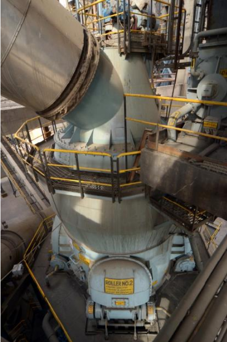
View of roller no. 2 of the LOESCHE mill type LM 43.4 D
