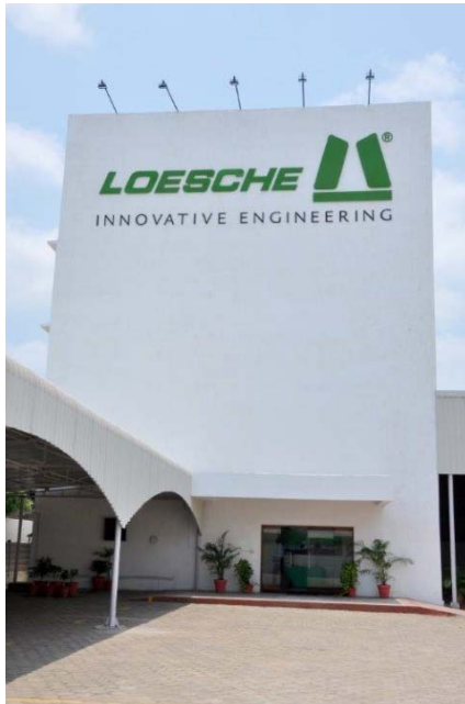
LOESCHE workshop in Chennai, India – office building
