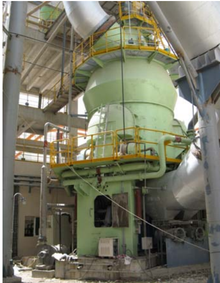
Similar mill type LM 35.3 D, Ras al Khaimah, United Arab Emirates
