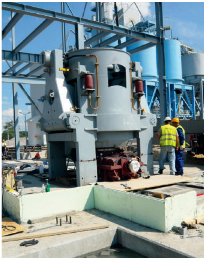
Loesche Mill type LM 15.200 under construction
